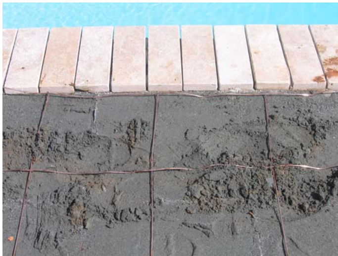
Figure 3: Installation of Equipotential Ground Mat
