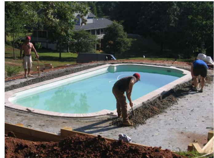
Figure 2: Installation of Ground Ring
